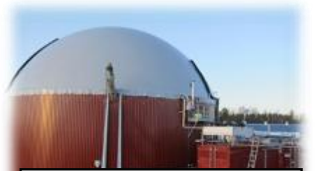
Hagelsrum 3 GWh (Drift operate since 2011)
