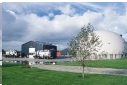
Thorso biogas plant, Denmark
