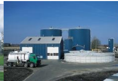
Studsgaard biogas plant, Denmark
