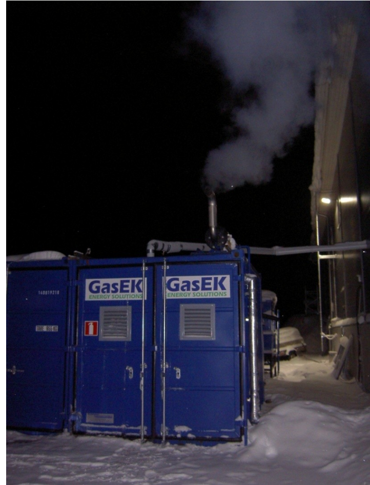
The woodgas container producing heat and electricity in winter (-35 °C)
