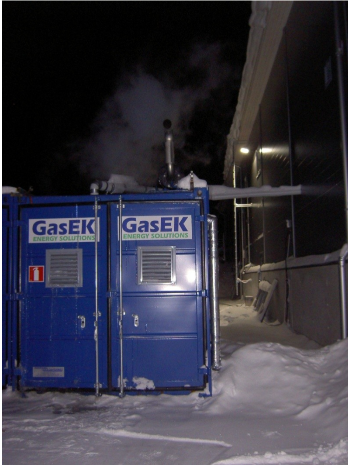
The woodgas container producing heat and electricity in winter (-35 °C)
