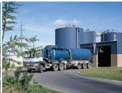
Ribe biogas plant, Denmark
