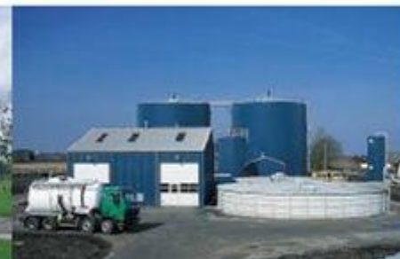
Studsgaard biogas plant, Denmark
