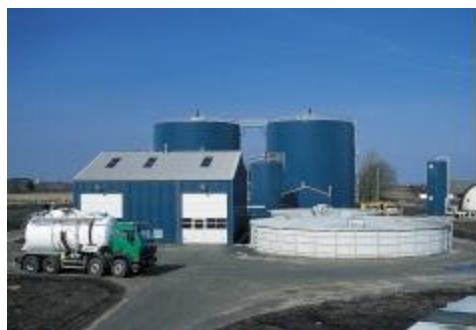
Studsgaard biogas plant, Denmark
