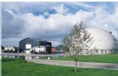
Thorso biogas plant, Denmark
