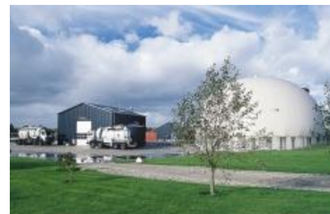
Thorso biogas plant, Denmark
