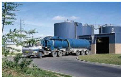
Ribe bioqas plant, Denmark
