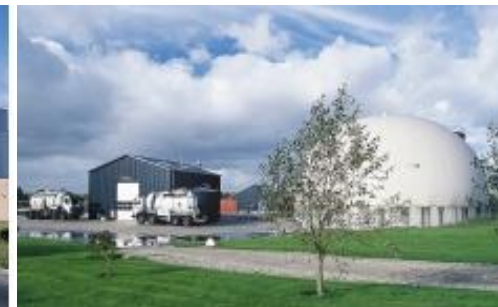
Thorso biogas plant, Denmark
