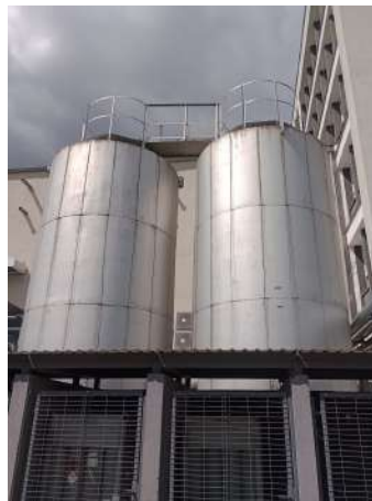
Fig. 13.15: Vacuum tanks.
