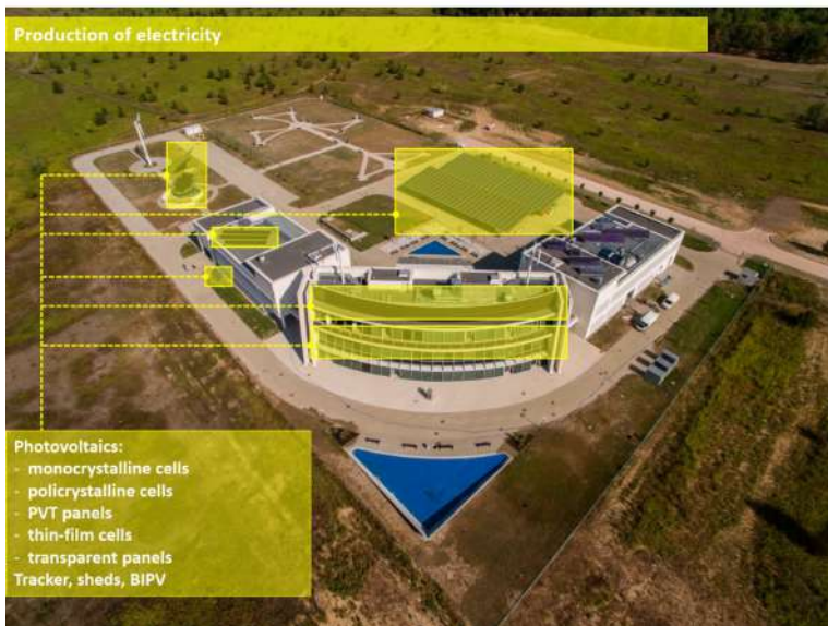
Production of electricity – equipment and its locations. source: Own materials.
