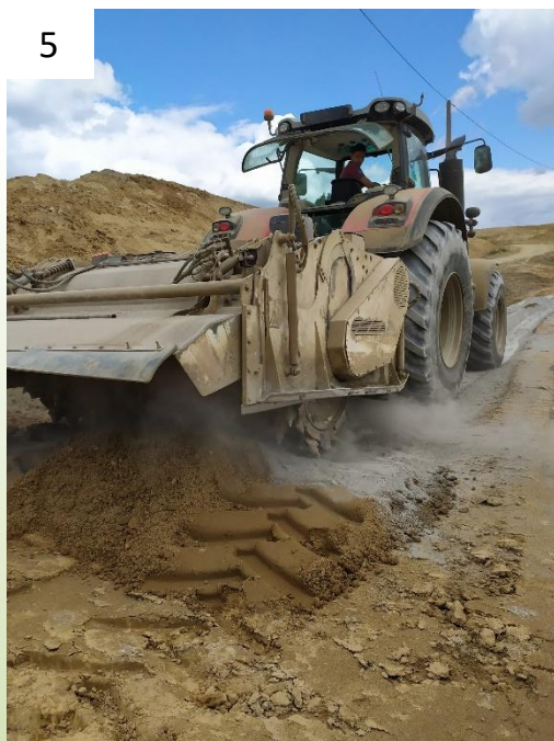
Mixing with the soil
