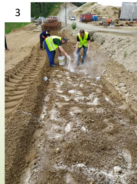
Implementation of 2 binding material
