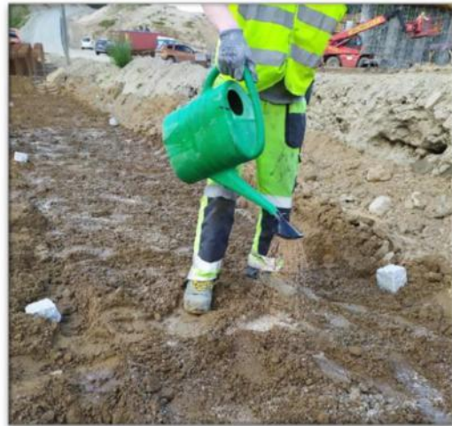
Fig. 2. Manual application of liquid soil stabilizers (emulsion based on plastic waste pyrolysis products - waxes).
