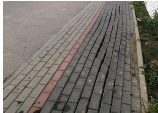
Fig. 1. Waste tires landfill and pavement damage due to unstable subsurface
